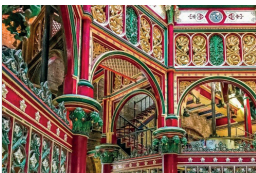
The Crossness Pumping Station
